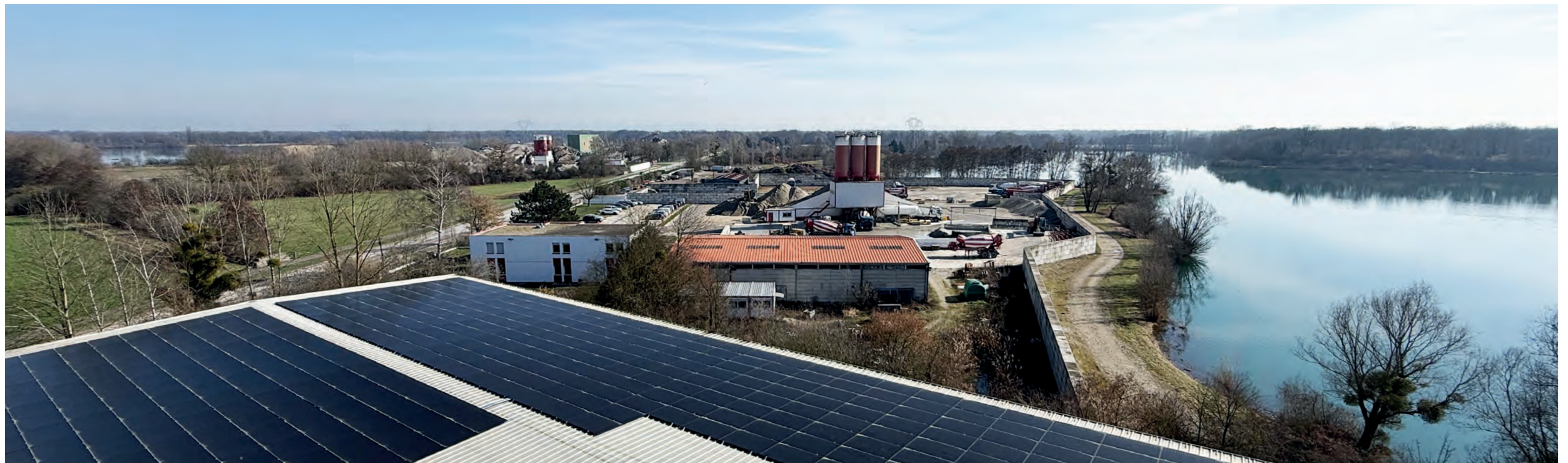
Photovoltaikmodule in Krautergersheim
